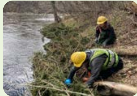
Cedar Tree Revetments
