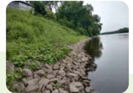
Riprap Toe + Vegetated Banks
