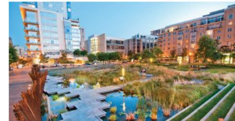
Urban Stormwater and amenity area
