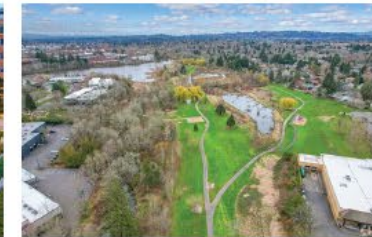
Naturalized stormwater and trail amenities
