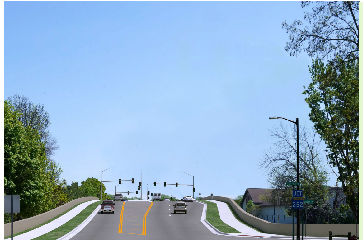
📍 Elevated crossroad severs the driveways near Hwy 252 from crossroad resulting in an inaccessible property.
