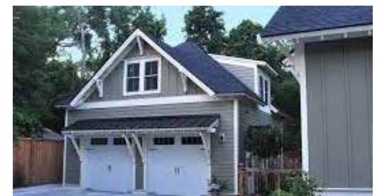
Attached to Accessory Structure
