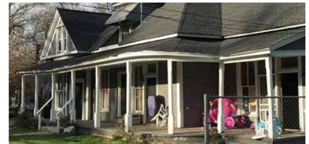
This structure is a 5-unit multiplex but could be a single-family home, or anything in between.
