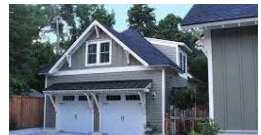
Attached to Accessory Structure
