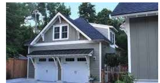
Attached to Accessory Structure
