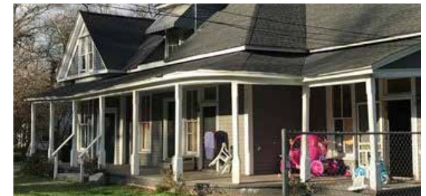
This structure is a 5-unit multiplex but could be a single-family home, or anything in between.
