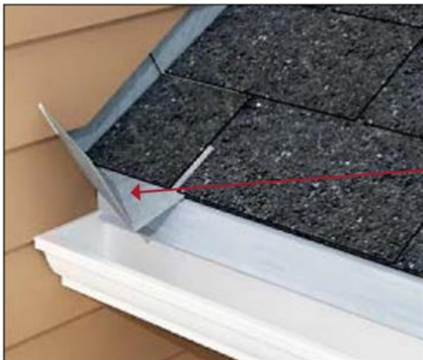
Kickout flashing
