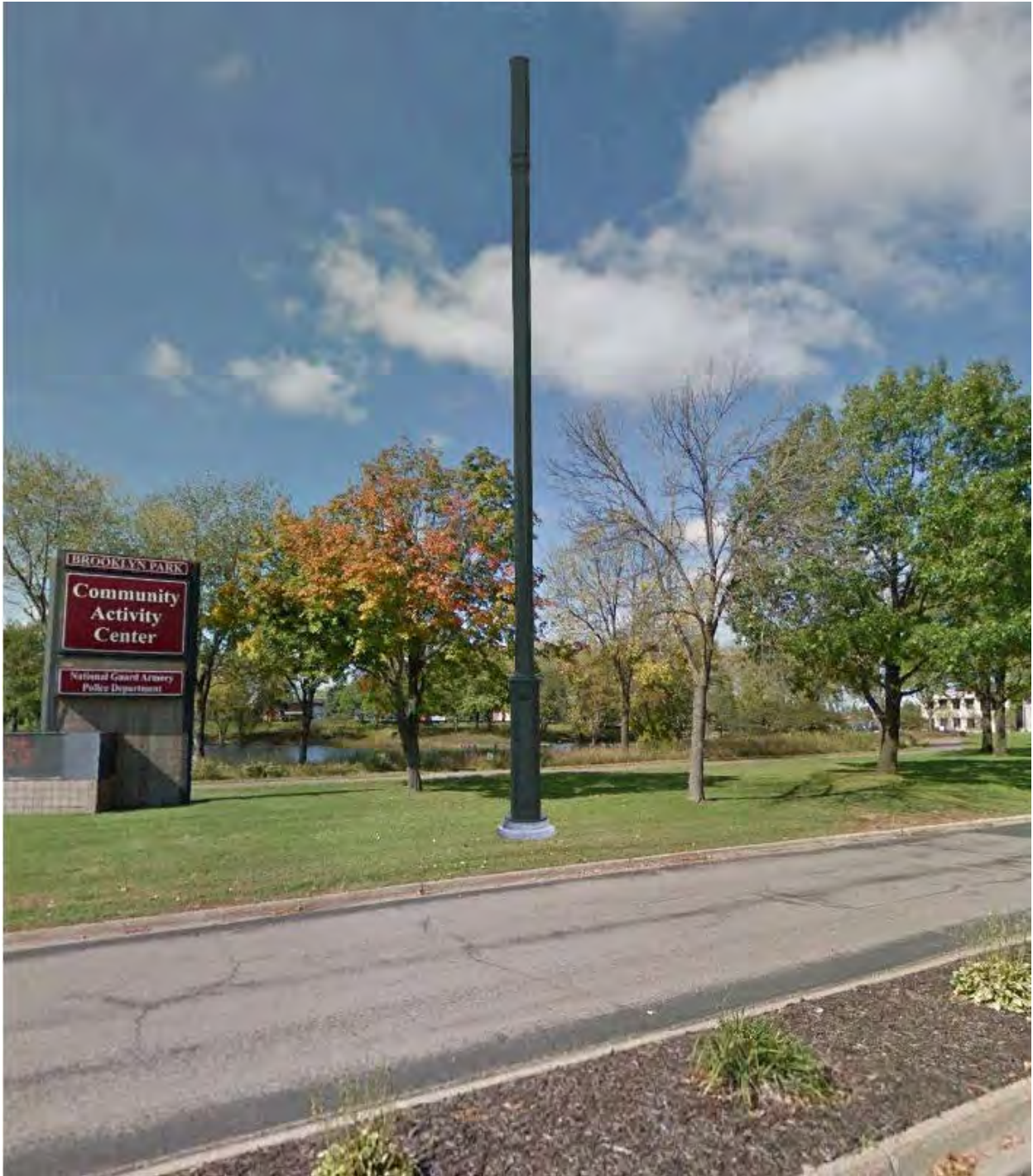
Figure 5-5: Picture of Freestanding Small Cell Assembly
