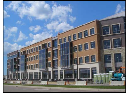
245,000 sq. ft Target office building
